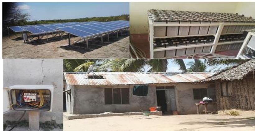
Fig. 2. Microgrid overview at Kisiju Pwani
