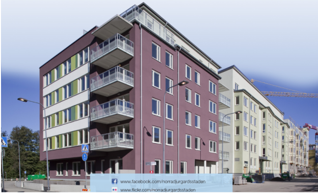
Fig. 1. An active apartment building in Royal Seaport project in Stockholm.
