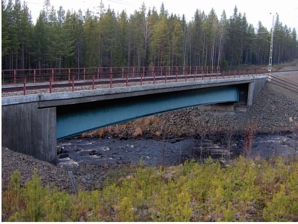
Figure 2: The bridge at Skidträsk.
