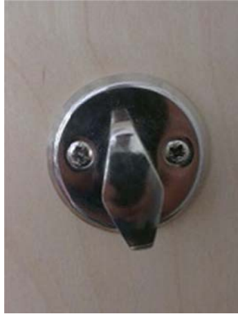
Figure 1-2: A latch to mechanically control the door lock on a door
