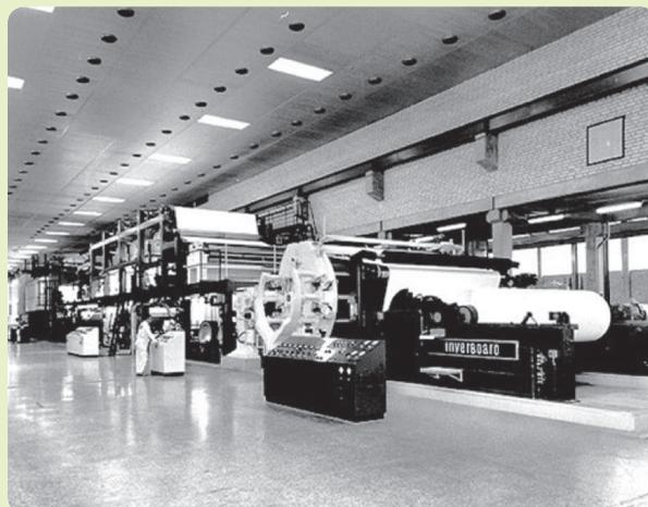
**FIGURE S3** Iggesund Paperboard's first cardboard machine (KM1) is still in use. However, it has been rebuilt several times since the photo was taken in 1968. The photo shows the reeling of the cardboard, and coating stations are in the middle of the picture. At the far left, the cardboard machine's drying unit is visible. (Source: Iggesund Paperboard; used with permission.)
