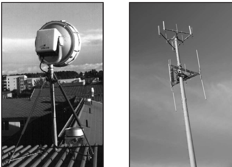
Figure 2.4: Left: Point-to-point microwave link, which connected the student dorm network in Linköping to the the campus network and the Internet, 1993–1996. Photo by Kjell Enblom, RydNet. Right: Cell phone tower in Oregon. Photo by Todd Klassy.
