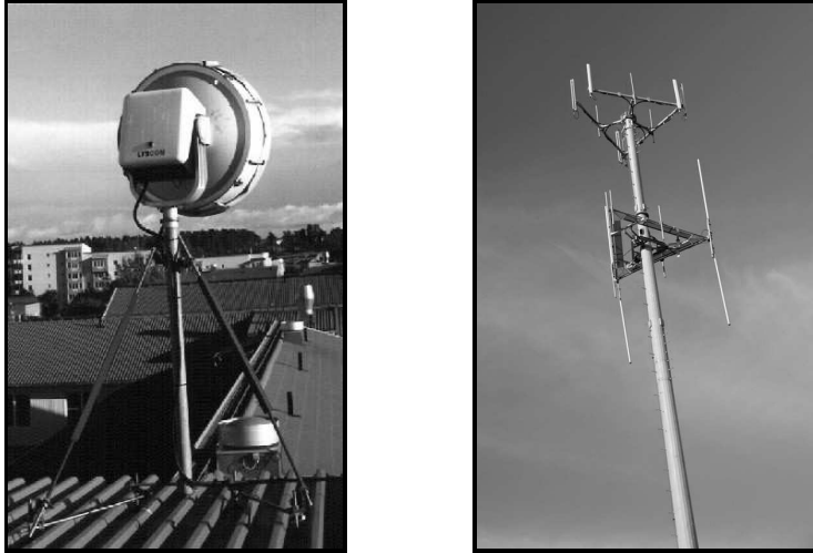
Figure 1.2: Left: Point-to-point microwave link, which connected the student dorm network in Linköping to the the campus network and the Internet, 1993–1996. Photo by Kjell Enblom, RydNet. Right: Cell phone tower in Oregon. Photo by Todd Klassy.
