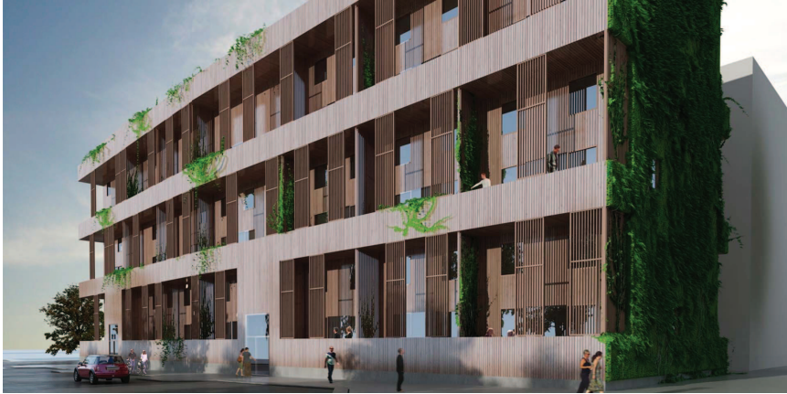
Figure 1.3: Wireless control is an important enabling technology for intelligent green buildings. The illustration shows a design project for the Stockholm Royal Seaport (courtesy of Folkhem & Wingårdh Architects).
